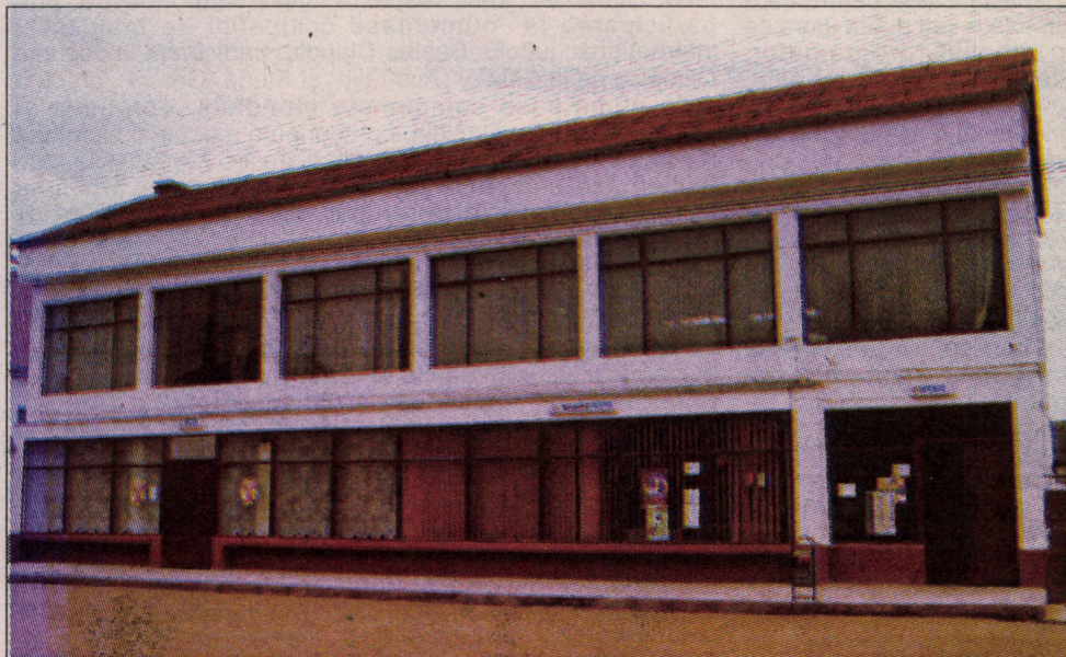
Complexul Comercial Alțâna
